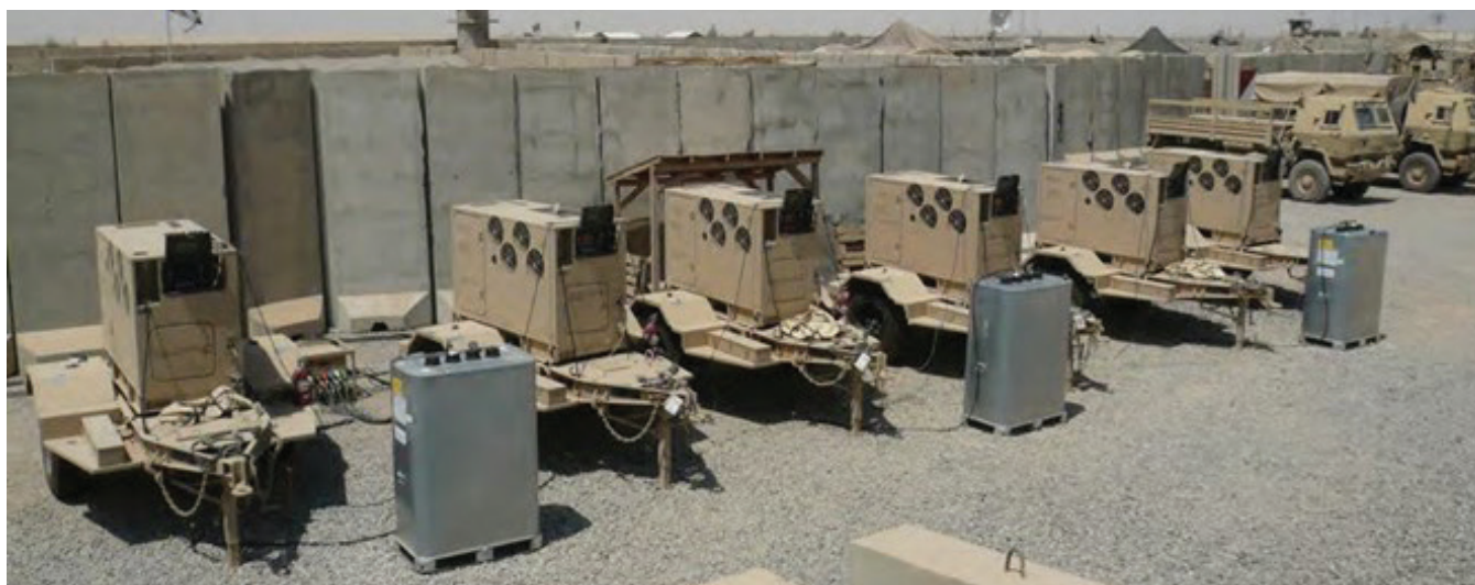
Figure 13. Operational Employment of an Advanced Medium Mobile Power Sources Microgrid (MG-5106 120 kW System), July 2018, Operation Inherent Resolve, U.S. Central Command Area of Responsibility
