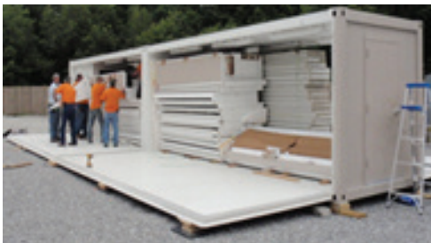
Panelized shelter (future): a reusable, transportable, simple, low-labor assembly, environmentally resilient, modular, and scalable shelter.
